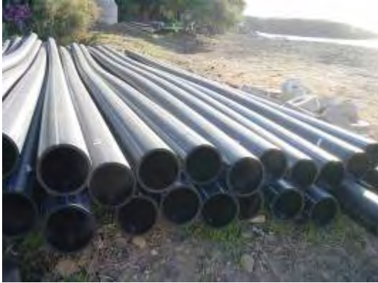
Fig. 16 Pipes joined on the shore
