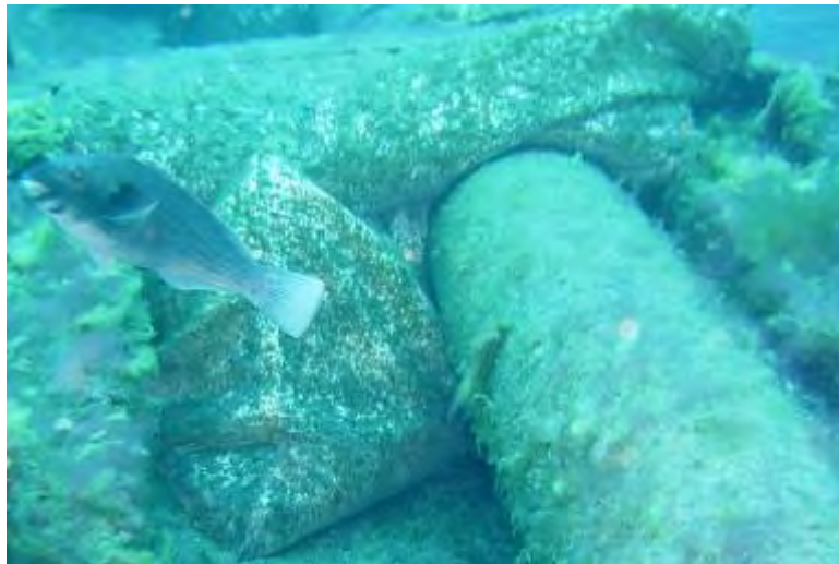
Fig. 2 Sand and concrete bags
