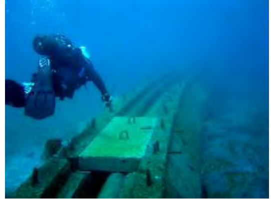
Fig. 17 Placing the pipe
