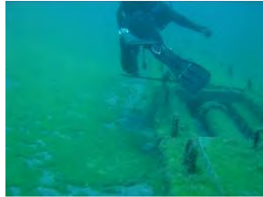
Fig. 11 Lifting caps while inspecting the emissary
