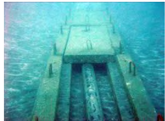
Fig. 19 Settling case ready for another inner pipe
