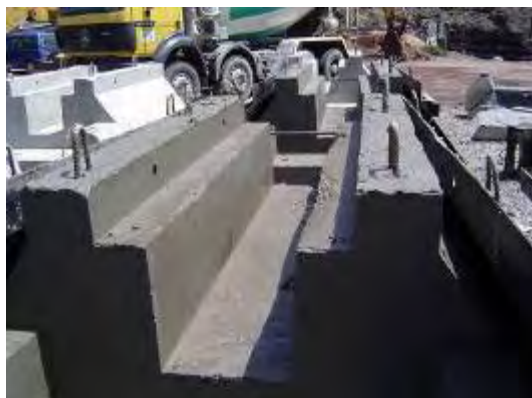
Fig. 14 Concreting of EMITE units
