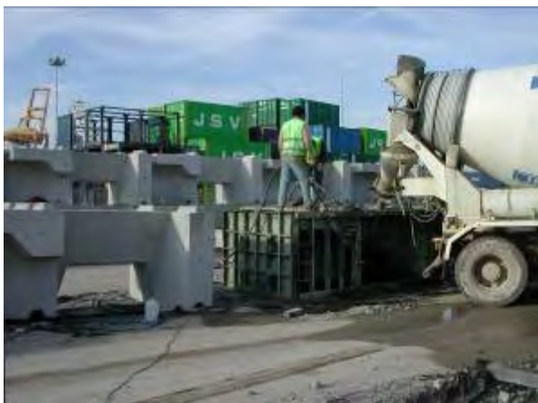
BARA unit, Concreting and transport of BARA units
