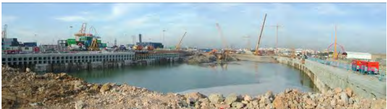
Construction of docks and port seawalls affected by waves
