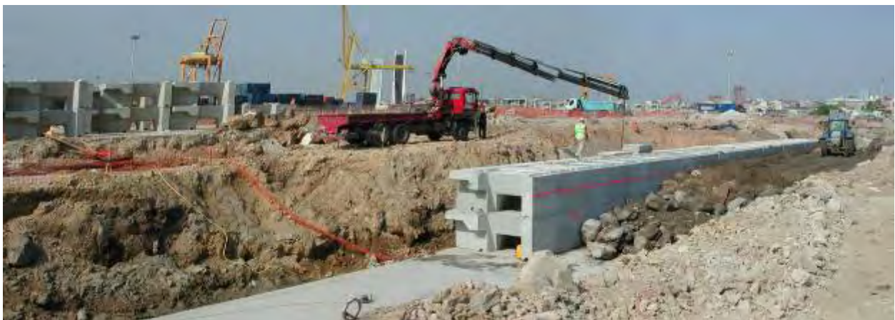
Filling materials on the structure's backside
