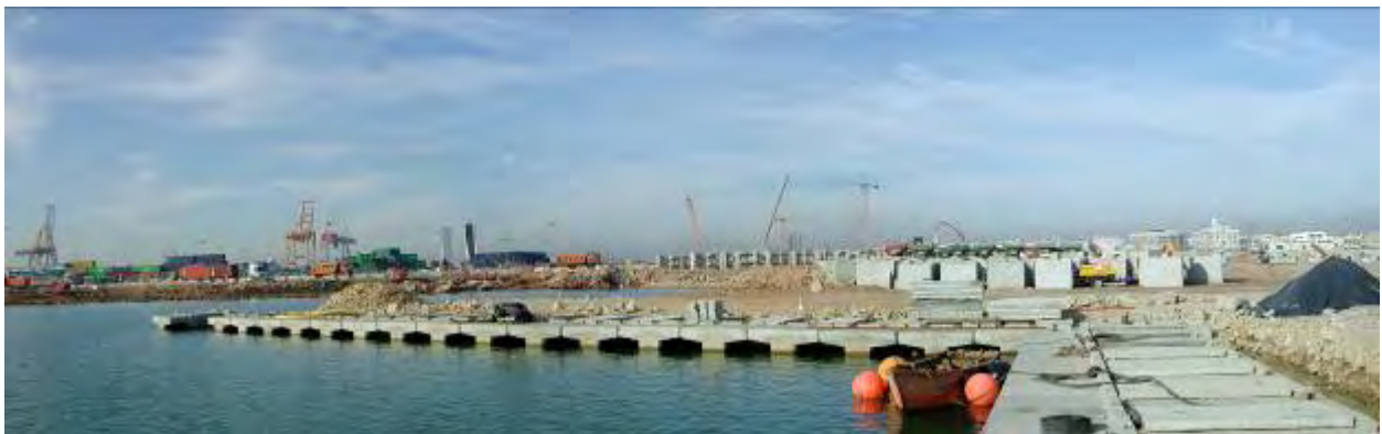
Superimpose placement of BARA unit
