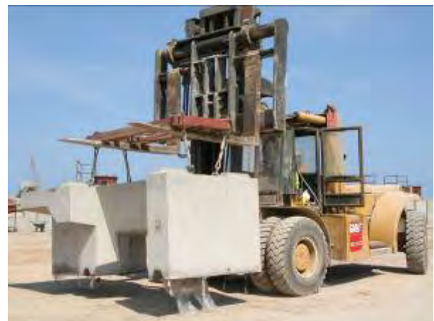
BARA unit, Concreting and transport of BARA units
